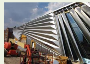
Construction of Broad Art Museum
